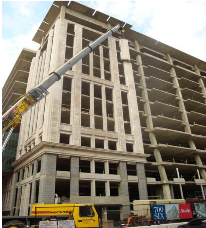
Picture 2.1-Concrete Superstructure
