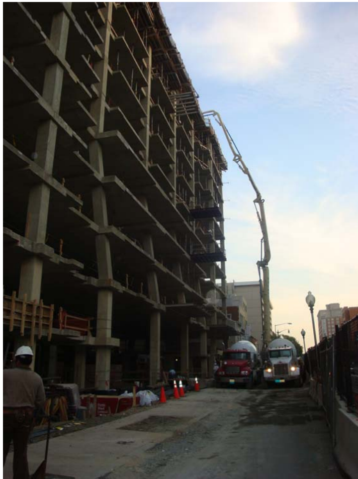
Picture 3.3-Concrete Pump Truck
