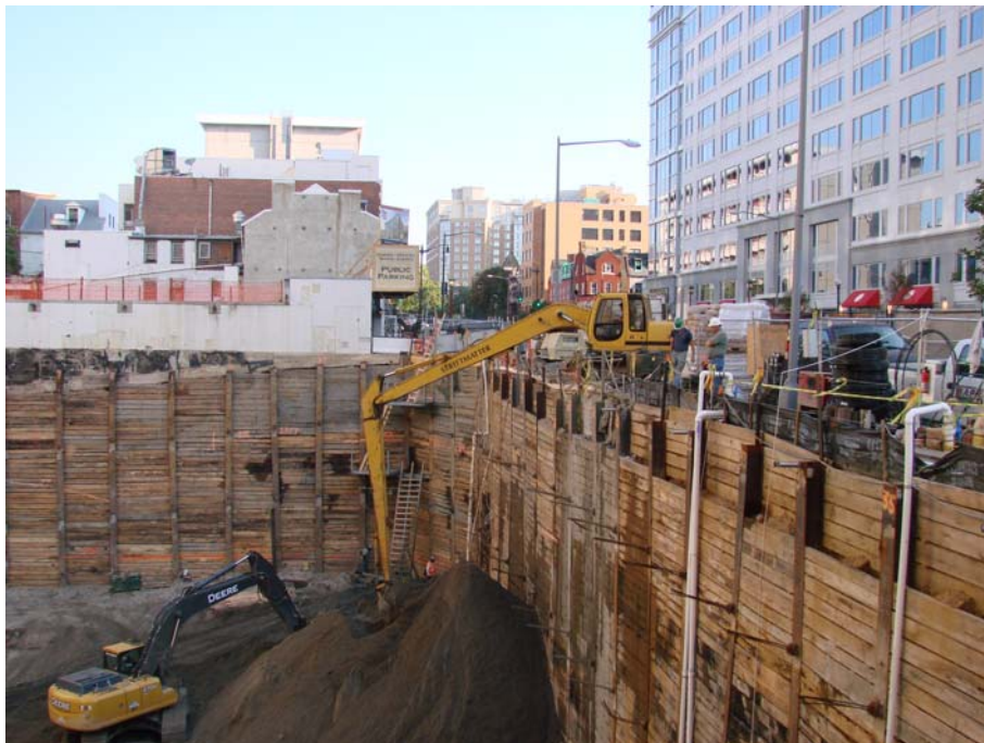
Picture 3.1 Extended Boom Excavator
